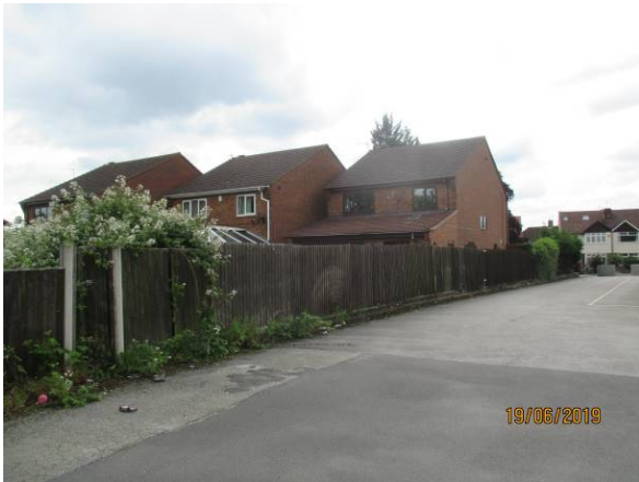
The rear elevations of 193, 195 and 197 Toton Lane
