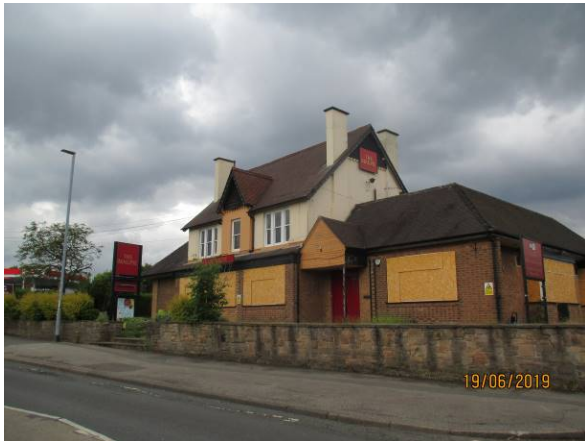
The Magpie PH, following closure and prior to demolition
